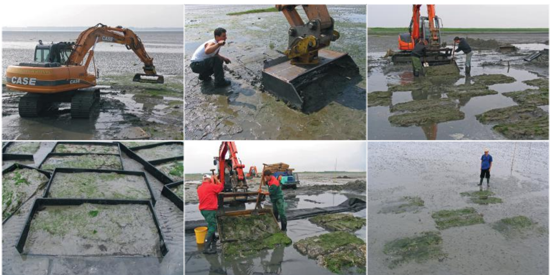
Plate 16. Photographic impression of the sod relocation method at the intertidal sites in the Eastern Scheldt, showing the modified backhoe scraping technique and transplant relocation.
