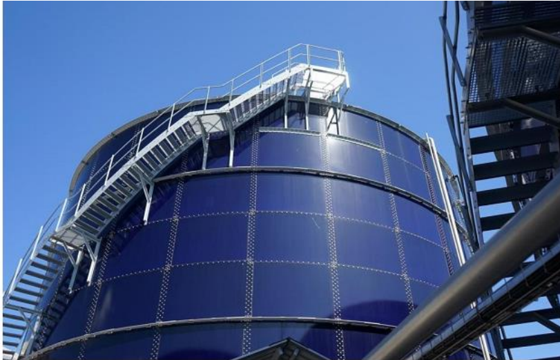
Operations will start at 30 percent by adding the necessary bacteria to the tanks (Thai Union) Photo License: CC-BY
